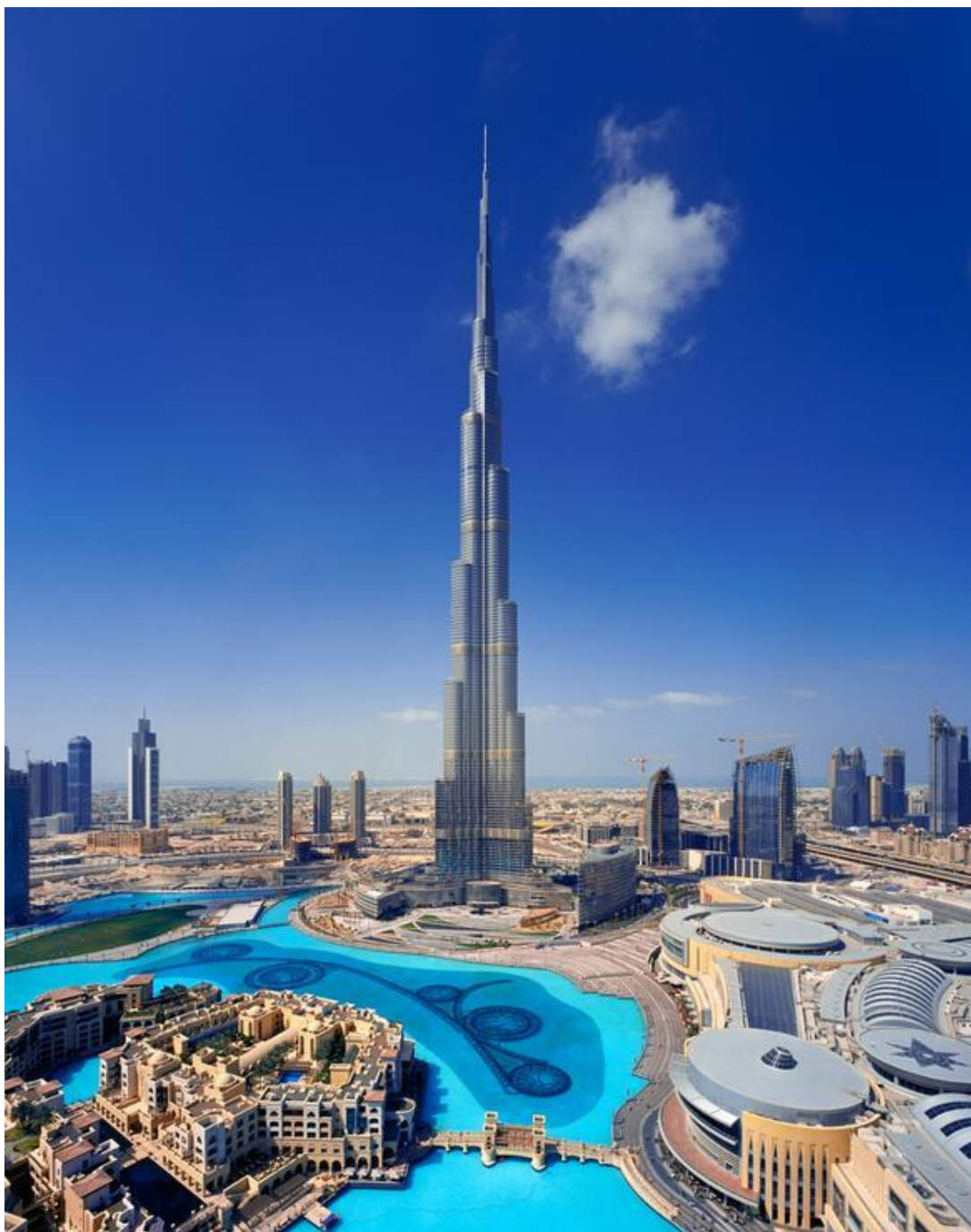
Ryc.99. arch. Adrian Smith & Skidmore, Owings and Merrill Burdż Chalif - Wieża Chalify , Dubaj (2004-2009r.)
