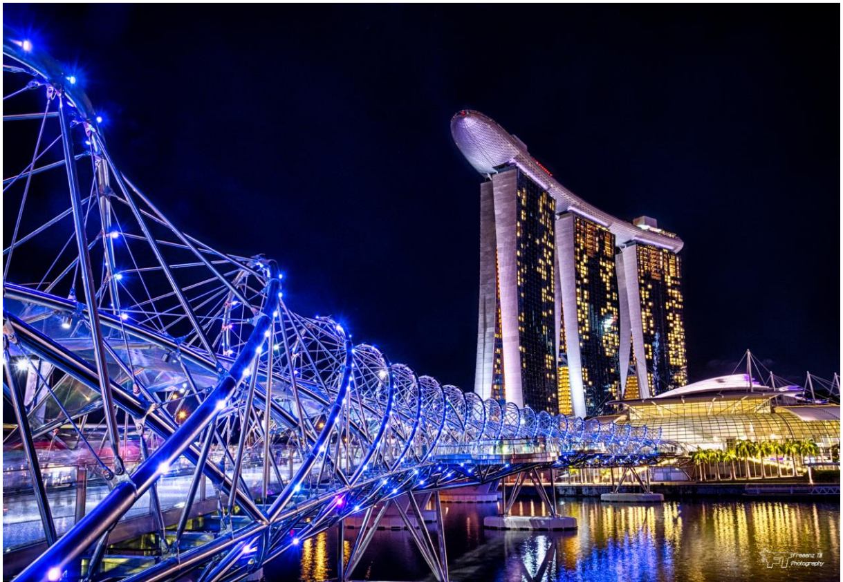
Ryc. 104 Helix Bridge & Hotel Marina Bay Sands w tle
