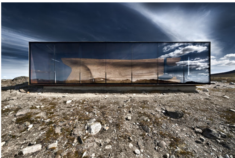
Ilu. 6.71 Schronisko Norwegian Wild Reindeer Pavilion by Snøhetta (Autor: Hunting Lodge by Snøhetta źródło: Int. 43)
